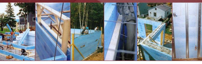
Rigid expanded polystyrene panels are ultralight, allowing easy moving and on-site handling. The 2 parallel panels that make up the insulating form are held together by tie rods to which the reinforcing steel bars are attached.
